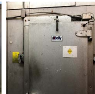
Walk-In Medium-Temperature Freezer
